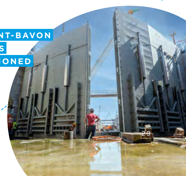
Installation of the lock gates of the Saint Bavon lock in Wielsbeke © De Vlaamse Waterweg
