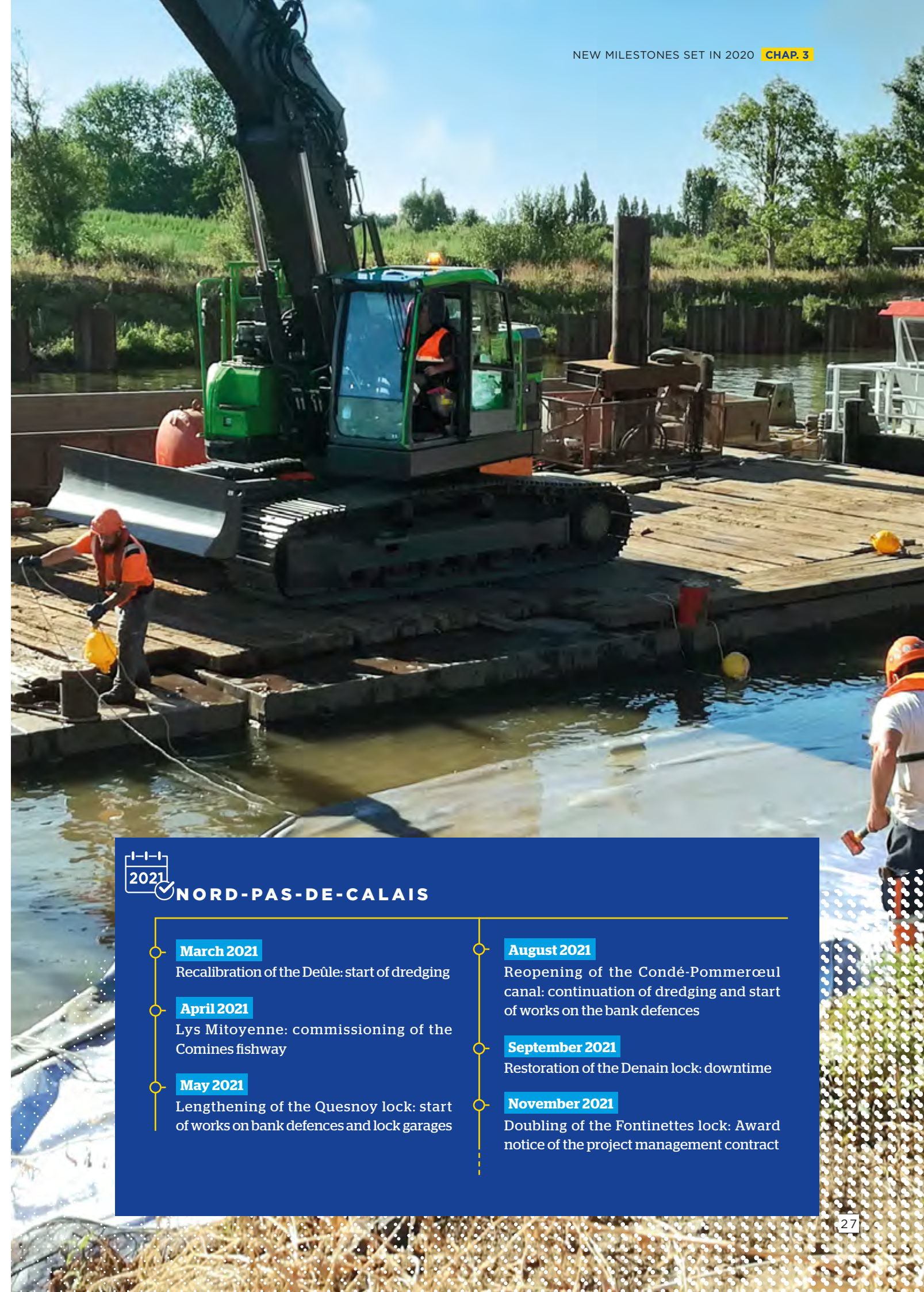
Lys recalibration - Securing geotextile on a slope before laying the riprap © VNF
